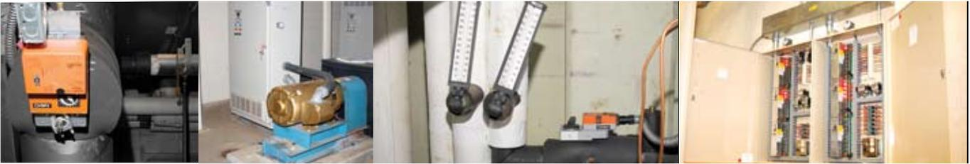
drives on the secondary and tertiary pumps and 2-way pressure independent valves at the cooling coils.
