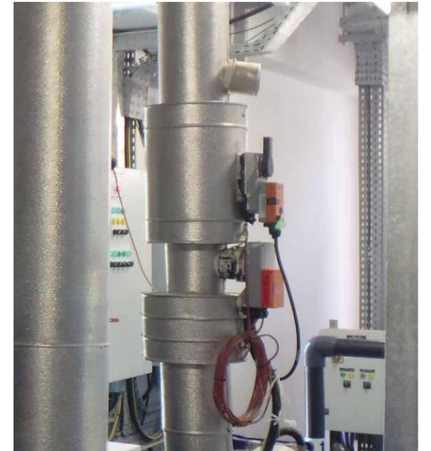
Figure 90: The supply of the Fancoil Units is equipped with the Belimo Energy Valve™
