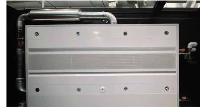
Figure 91: Ceiling integrated chilled beam with air and chilled water supply
