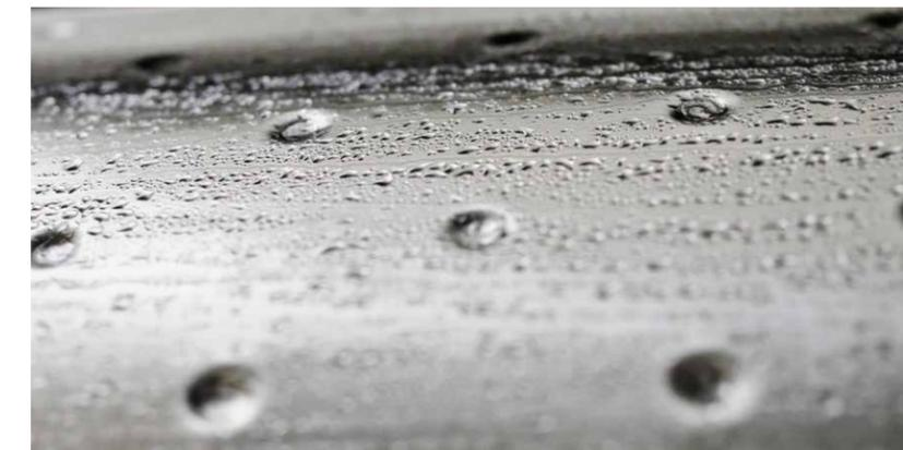
Figure 95: Condensation of humid air on the cold coil surface. The supplied cooling water needs to be above indoor dew point to prevent condensation
