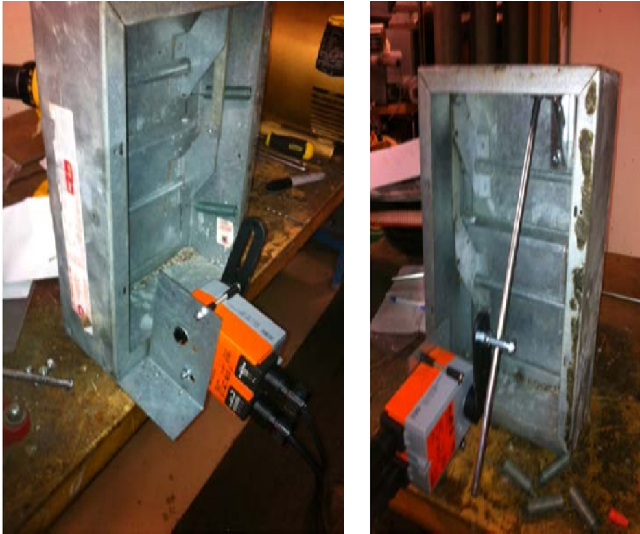
COMPLETED INSTALLATION OF FSTF120
