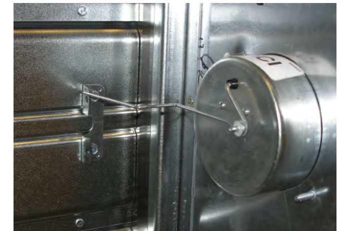
Figure 2. Typical damper position indication switch assembly. Image courtesy of Greenheck.
