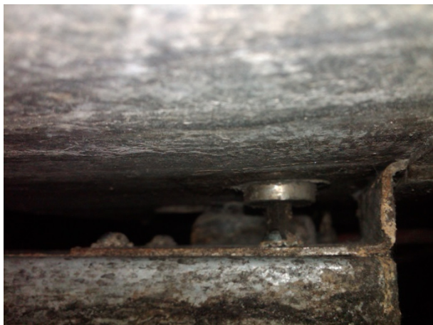
Detail of duct, hub, shaft, and motor.
