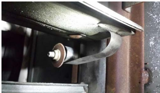
FUNCTIONAL Negator spring connecting post and damper blade.
