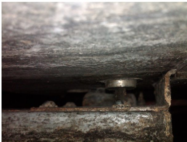
Detail of duct, hub, shaft, and motor.
