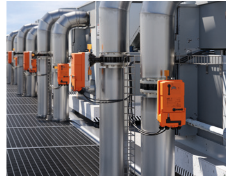
Butterfly valves with JR actuators
