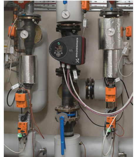
Shunt group with Belimo Energy Valves™ built on site.
