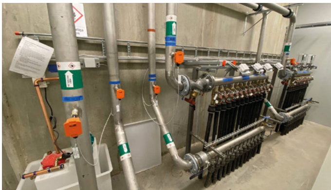
Energy supply from a geothermal source with built-in energy storage for heating and cooling and a backup connection to the district heating system.
