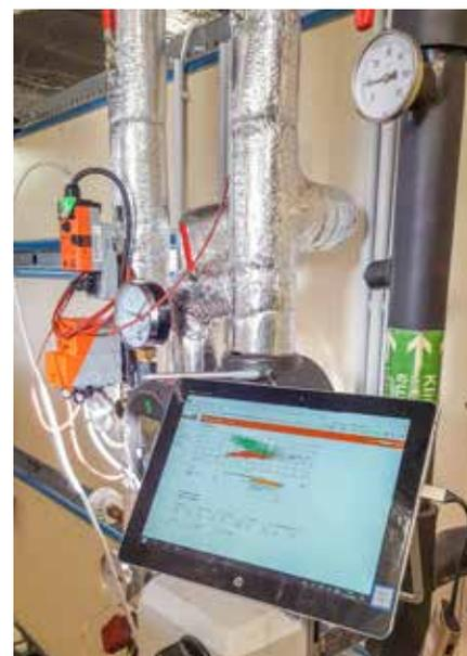
Evaluation of the recorded data to optimise delta T and the  $V_{max}$  value in the roof ventilation centre.
